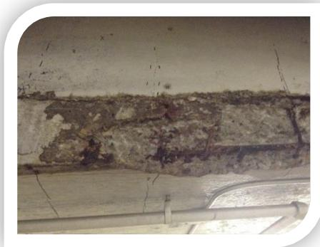
In 2015 Maverick was involved in a project in Edmonton. A concrete parkade ramp had been damaged by water and freeze/thaw cycles. Engineers were working on a solution, but had no existing drawings or references which explained how the ramp had been built originally.
